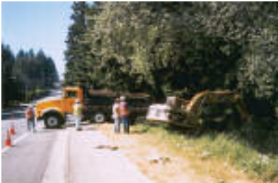
Trackhoe in the ditch at 24th NE
